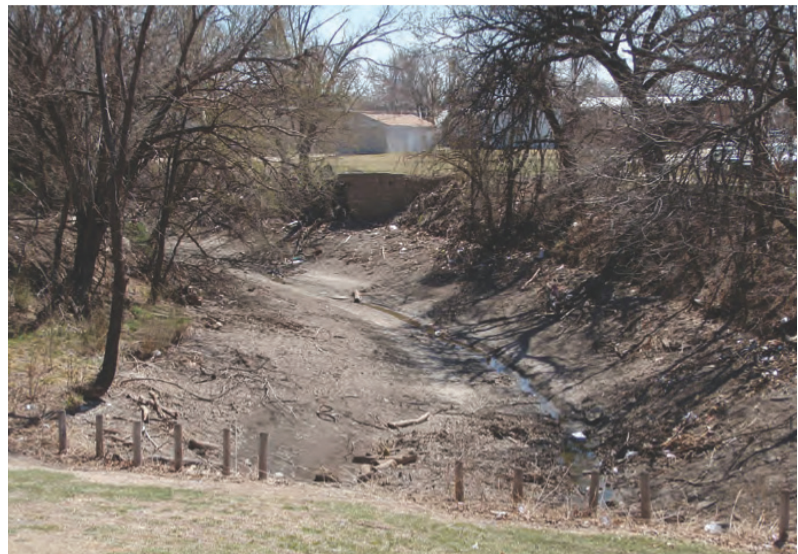
Existing Dry Channel
